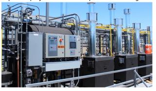
Figure 2, Control Panel Exterior. The HMI interface provides intuitive control and monitoring of the boiler system.
