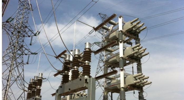
*You'll note that these capacitors above are connected in series. A phase and neutral line is connected to each capacitor so that it can fulfill its role of correcting the power factor of the system. Although a capacitor bank plays a crucial role in a substation there are some drawbacks associated with their use.*
